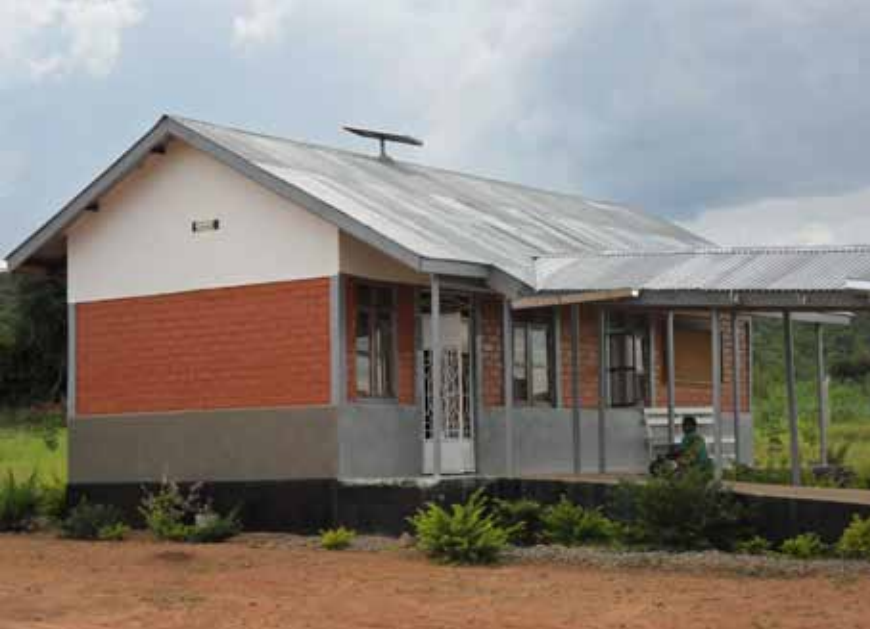
Figure 4.2: Solar Electrified Clinic Mbola
