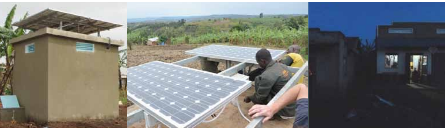
Figure 9.1, SharedSolar, (left to right): a shed housing the batteries and electronics; solar panel installation; home with electric lights powered by SharedSolar next to a home using kerosene lighting
