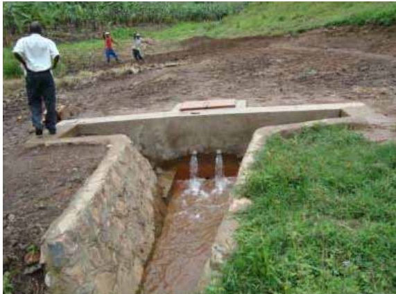
Figure 9.9: Protection of Ruhiira's water source
