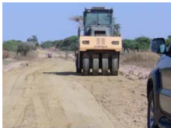
Figure 7.8: Road construction in the Potou cluster
