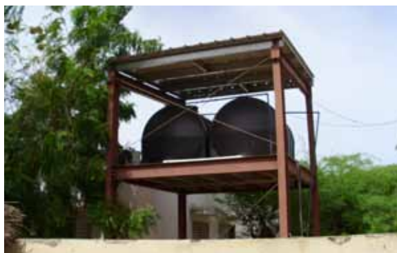
Figure 4.5: Health Clinic Water Storage Tanks; Potou, Senegal
