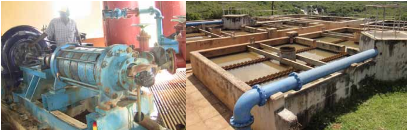
Figure 8.13: The Sidindi-Malanga project: turbine to be rehabilitated at Yala River intake (left); water treatment plant in Nyamninia Village (right).
