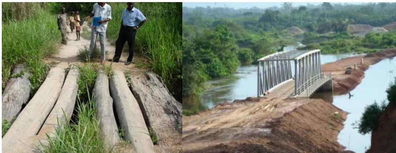
Figure 6.11: A wooden culvert that was replaced by concrete ring (left); a steel bridge installed by the government (right).
