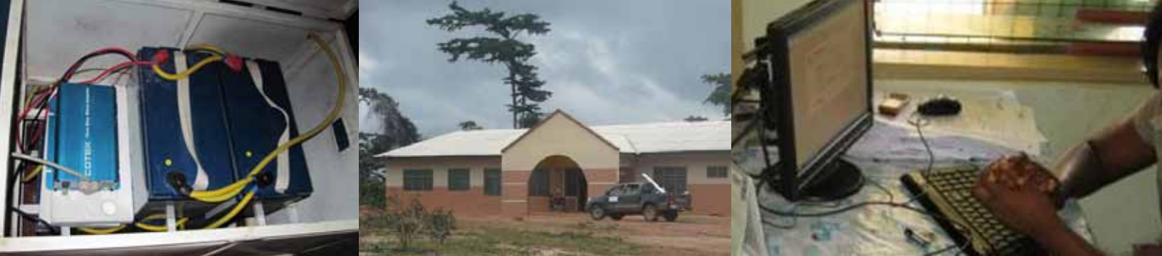
Figure 6.6 (left to right): a battery and inverter at Watreso Clinic; the newly built, grid-connected Assamang Clinic; a low-wattage computer used by a community health worker.
