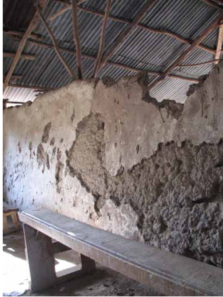
Dilapidated school, since replaced by MVP, in Sauri, Kenya
