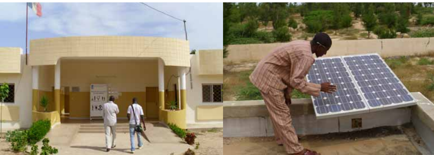
Figure 7.3: The grid electrified Rural Council Building (left); solar installation at Fishery Post (right)
