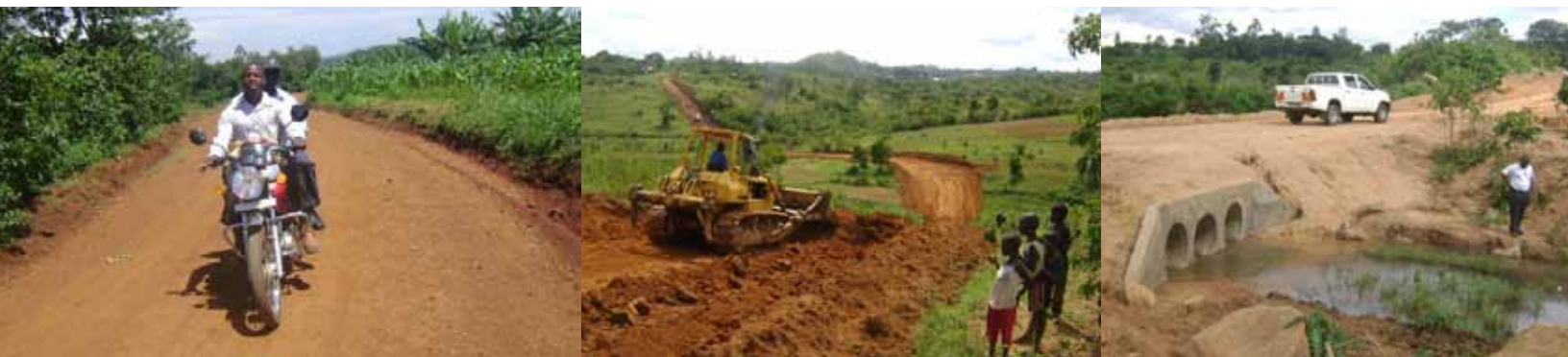
Figure 8.10: (left to right) Rehabilitated Saola Road in Jina Village, Rawalo-Madangala Road construction, Culverts at Muhanda-Arude Road
