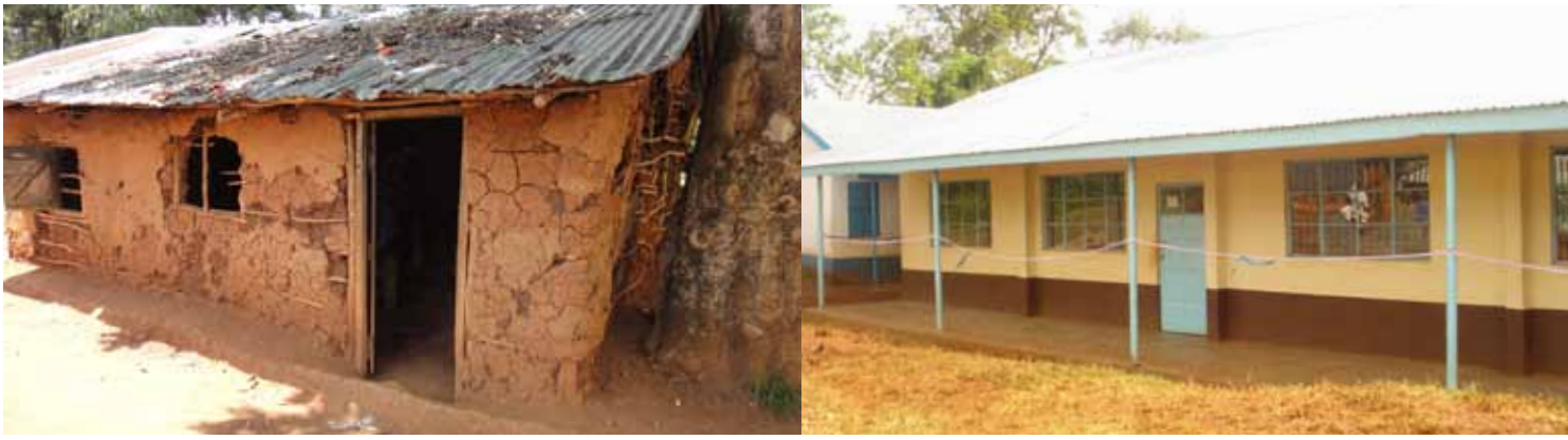
Figure 8.5: Uyonga Primary School (before (left) and after construction (right))
