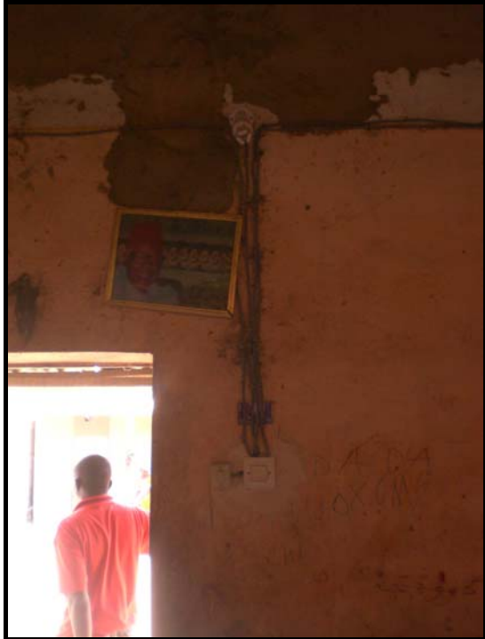
Picture 43: Electric Installation inside a shop
