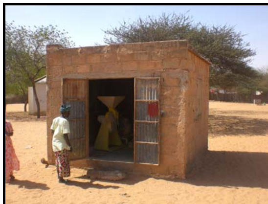
Picture 89: Shelter for the grinding mill in Whakhaldjiam.
