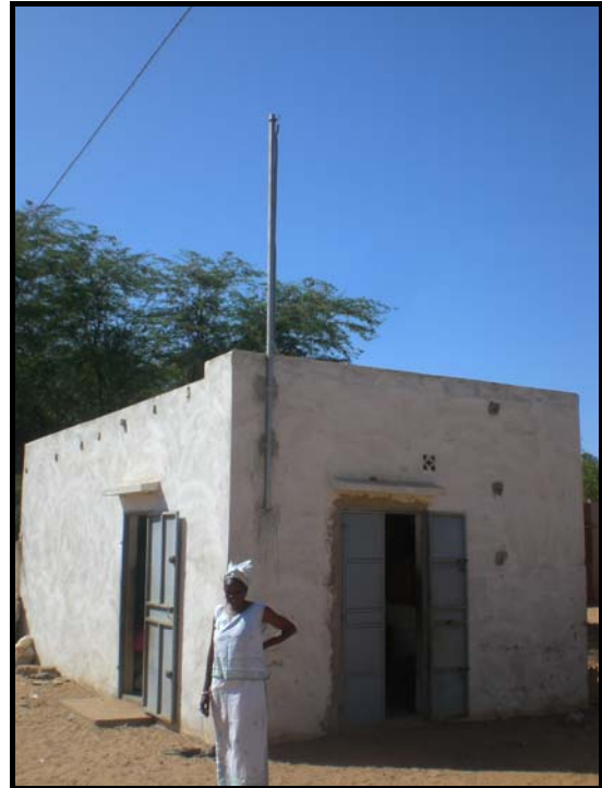
Picture 65: Pole installed for the connection to the grid
