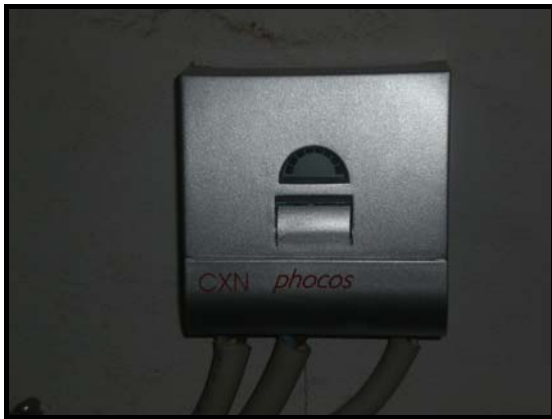
Picture 4: Charge Controller
