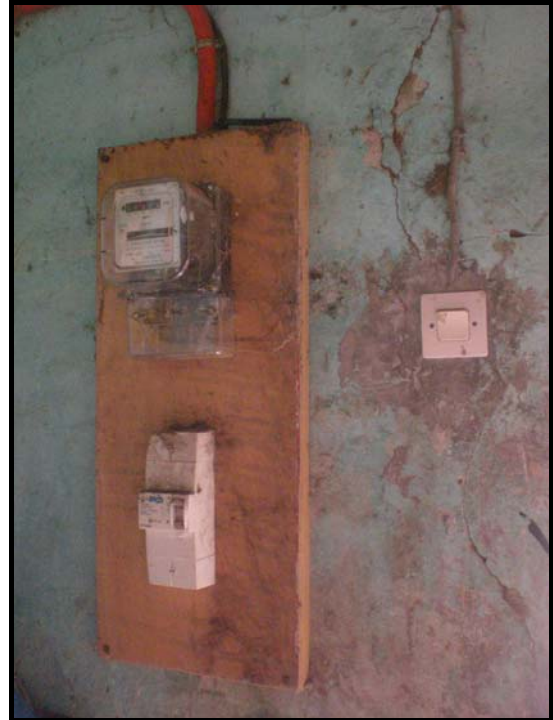
Picture 44: Electricity meter
