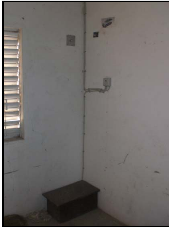
Picture 8: Battery and charge controller
