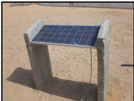
Picture 33: PV solar module
