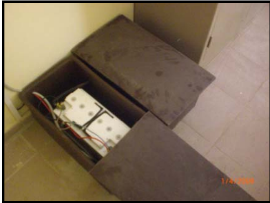
Picture 38: Batteries in the Fishing Post
