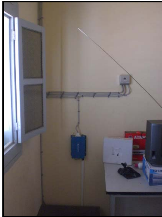
Picture 26: Inverter and controller
