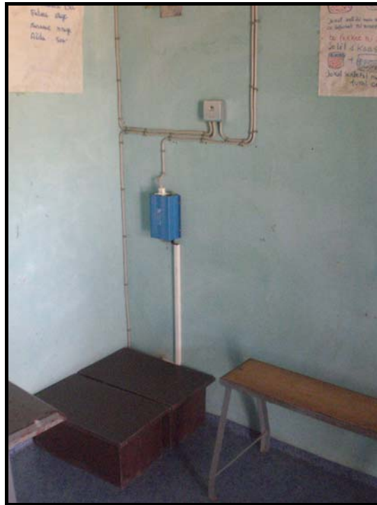
Picture 29: Batteries, Inverter and Controller
