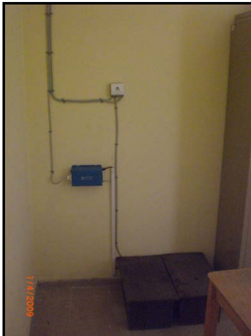
Picture 40: Batteries, inverter and controller in the Fishing Post
