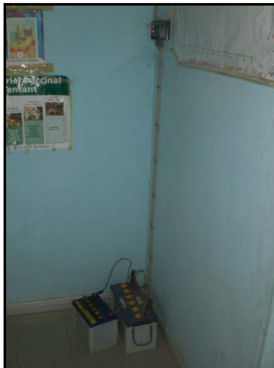
Picture 32: Batteries and controller
