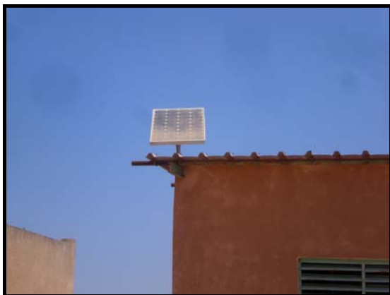
Picture 6: PV Solar module, 75Wc
